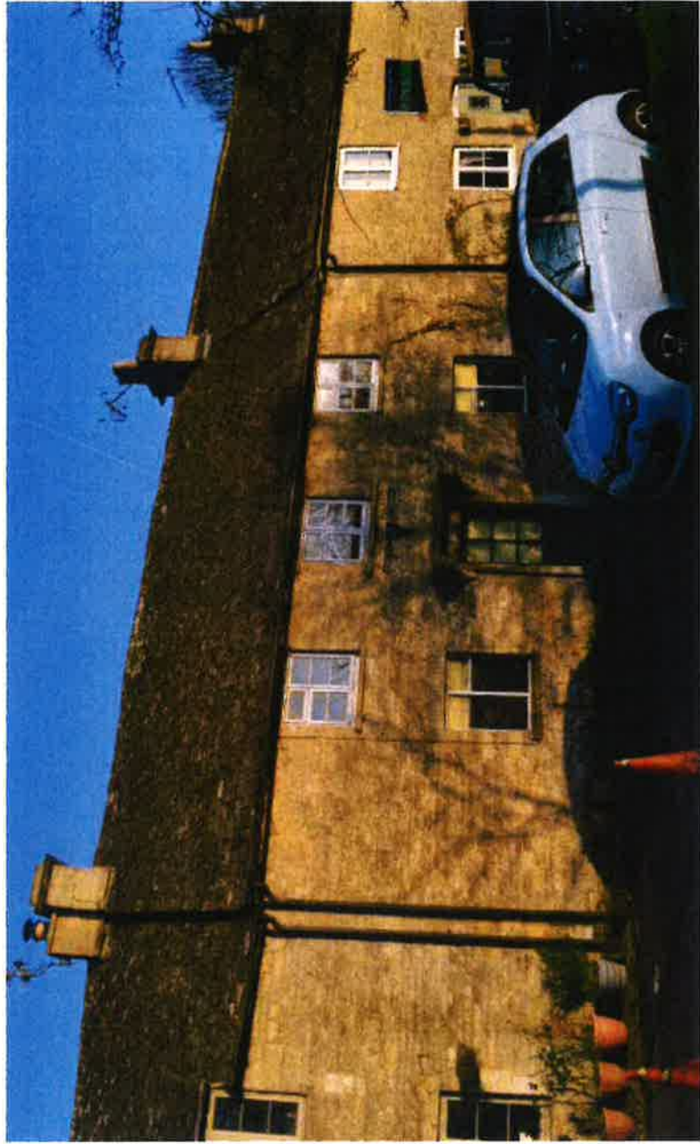
Fig 11: Front elevation showing central door canopy and replacement windows.
