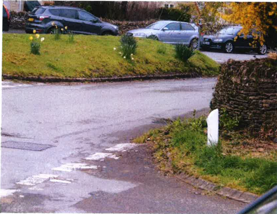
DRIVERS VIEW SOUTHBOUND OF BLIND EXIT FROM BACK LANE ONTO THE POUND & VILLAGE STREET
